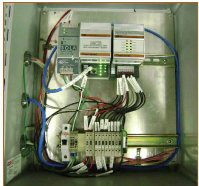
Figure 3. The local node of the communications system developed for the Devil's Tower platform interfaces with a remote node to provide an integrated system for communicating potential problems between the control rooms of a control ship and the oil platform. The local node communicates with a network mode through the use of an Ethernet network and the NET Concentrator System (NCS) Distributed I/O data concentrator solution; local and remote consoles allow operators to take action should a problem be detected.
