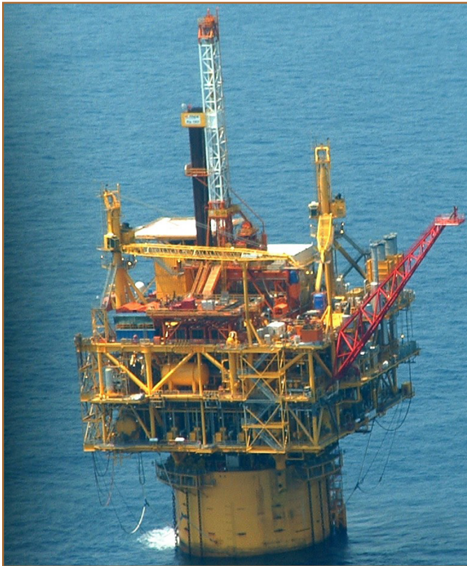
Figure 1. Rising more than one mile above the ocean floor, the Devil's Tower oil platform is one of the largest in the Gulf Coast.
