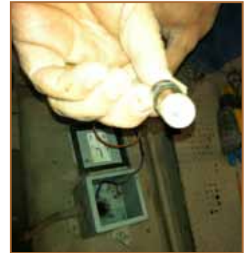
Figure 2. The older, non-contact I/R sensors which had previously been used at the mine. Because they were unable to get close to the ball bearings, they could only measure the ambient temperature near the bearing.
