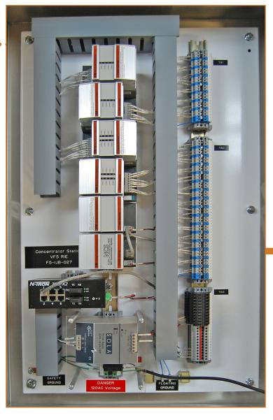
The control room modules output 4-20mA and discrete or relay output signals, which are wired into the control system's I/O cards
