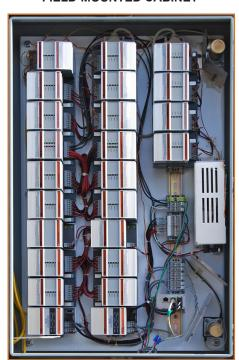
The instruments are wired into an input module in the field, which connects via a single twisted pair to a peer module in the control room.
