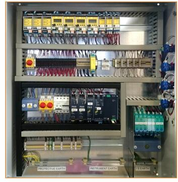
Our wide assortment of high-density instruments allow a modular approach to system design. We can install just one, a few, or hundreds of our DIN-style or plug-in instruments inside a standard or customized panel of your choosing.
