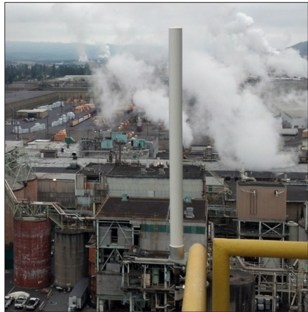
Figure 2. The omnidirectional antenna situated on the boiler room rooftop offers complete radio signal coverage for the entire site.
