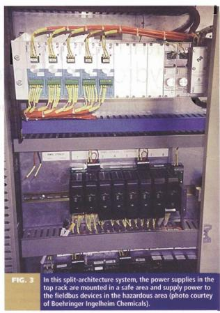
known as Fieldbus Intrinsically Safe Concept (FISCO), whereby they established experimentally that a nonlinear current-limited power supply could be used to extend the allowable current and, hence, effectively drive more devices in a hazardous area. FISCO power supplies are available that can deliver 110 mA into IIC/ Group A/B-rated hazardous areas driving, say, six devices. Fig. 2B shows a FISCO segment configuration.
