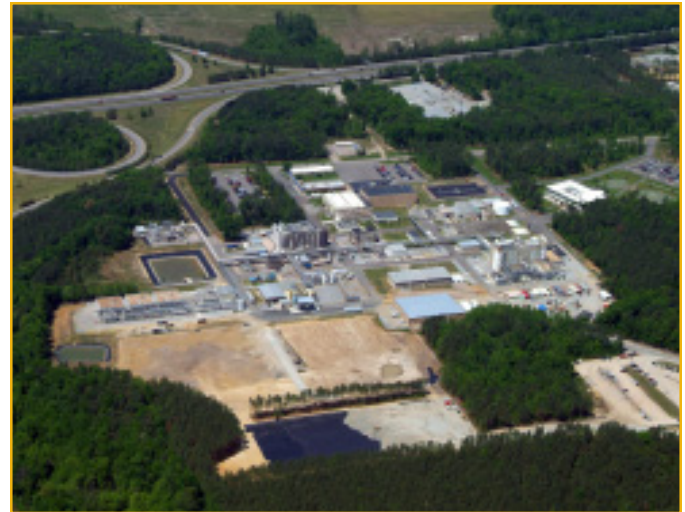
Production areas at Boehringer Ingelheim Chemicals plant in Petersburg, VA, are deemed hazardous, requiring an intrinsically safe fieldbus installation.
